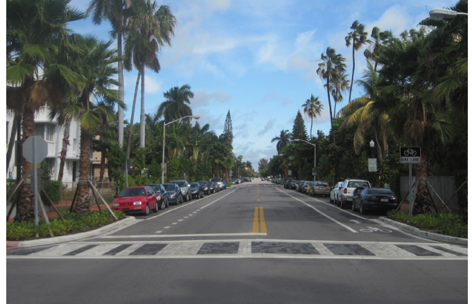
A short segment of Euclid Avenue now includes bicycle lanes, curb extensions/rain gardens, and enhanced crosswalks.
