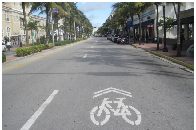
Sharrows on Washington Ave. help guide bicyclists away from the opening doors of parked cars. They also indicate to motorists that the road is a shared space.
