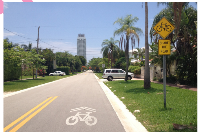
East-west and north-south bicycle lanes and shared use lane markings (sharrows, pictured above) are commonly found in the Nautilus neighborhood.
