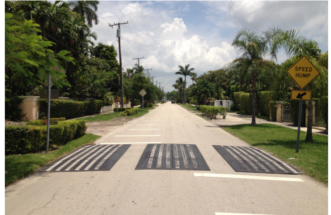
On North Bay Road, which provides a north-south alternative to Alton Road, thick rubber speed humps leave gaps where cyclists may travel unimpeded.
