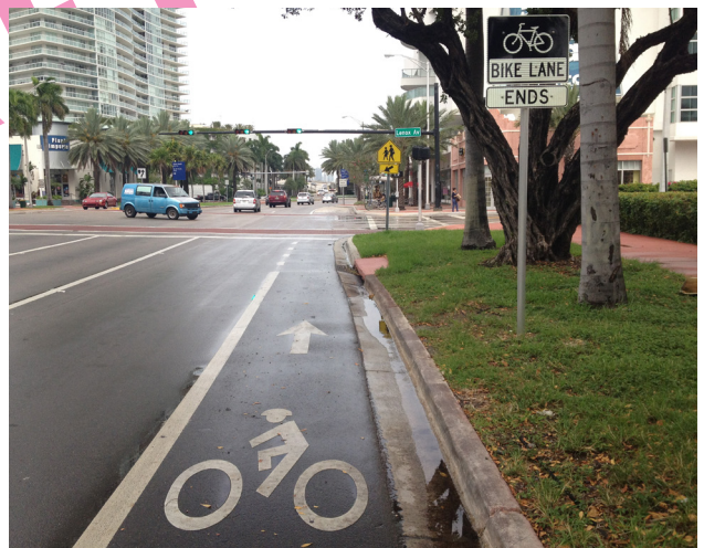
New bicycle lanes along 5th St. improve conditions for skilled bicyclists. However, the eastbound lane ends suddenly at Lenox Street, and without indication for how cyclists should continue to navigate.
